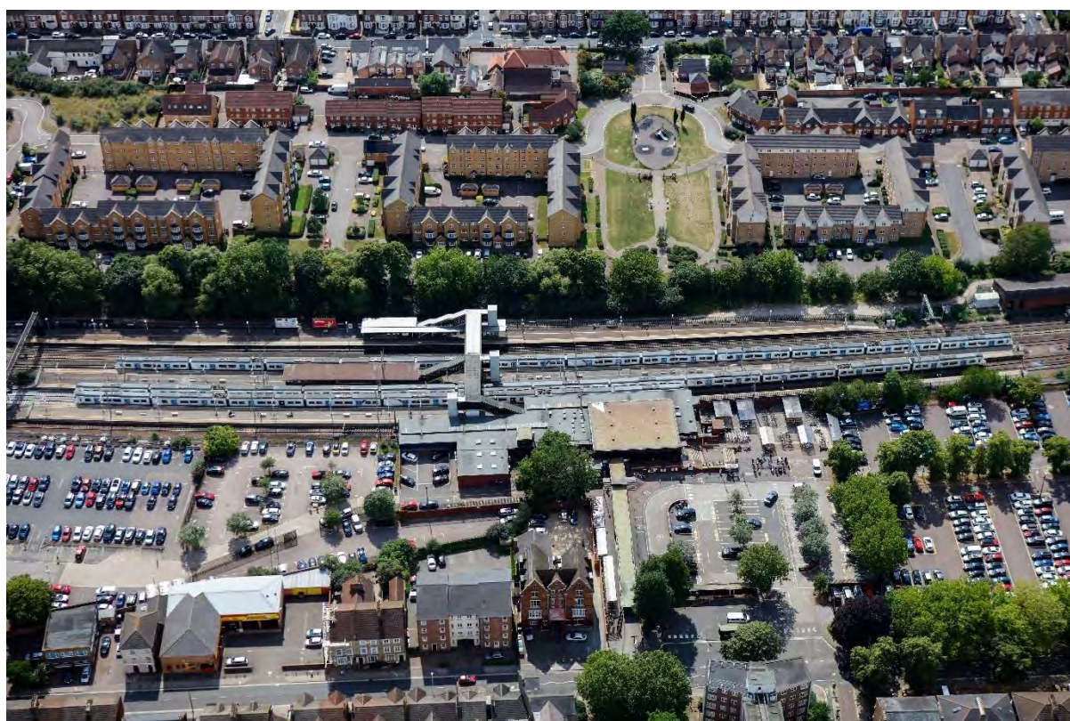
Figure 1-8: Bedford Midland Station
